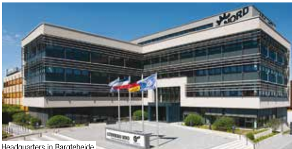
Headquarters in Bargteheide
