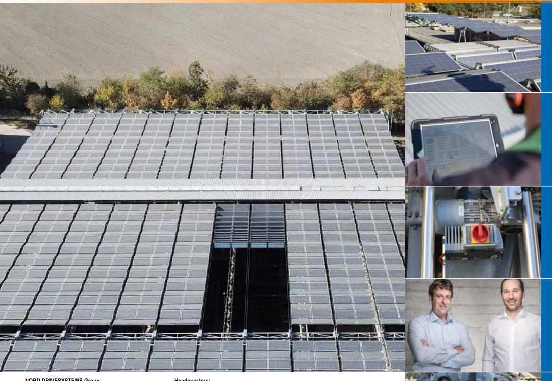
**World's first solar folding** roof over a sewage treatment plant
